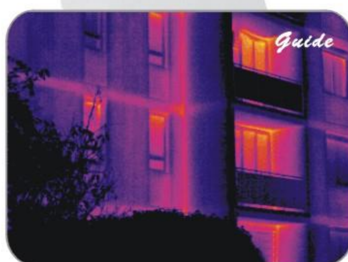
Inspect building structure
